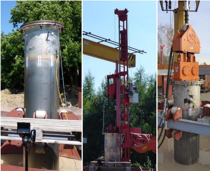
**Figure 5-14: Pile before installation (left), during impact driving (middle) and during vibratory driving (right)**
