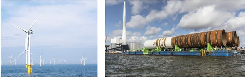
**Figure 1 : (left) The Nobelwind offshore wind farm is the most recent offshore wind farm in Belgium on monopile foundations. (right) Monopiles for the Horns rev 3 wind farm, modern day monopiles are relatively short with large diameters [Offshorewind.biz,2017]**
