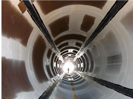
**Figure 3 : Monopile of the Nobelwind offshore wind farm after installation of the four optical fiber lines**
