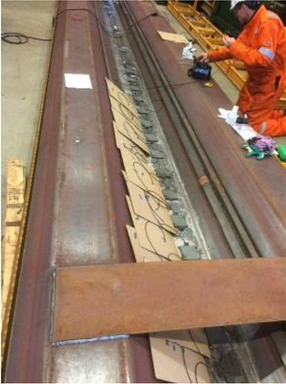
**Fig. 7: Installation of the sensors on a sheetpile. The sensing elements are covered with an individual protective cover which does not interfere with their function as strain sensors.**
