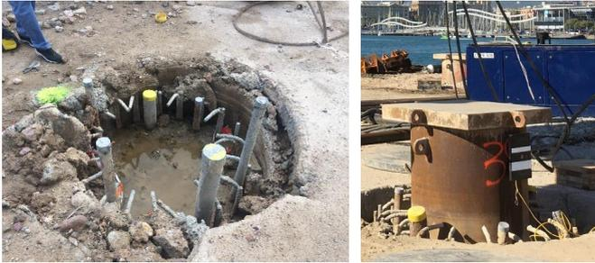
**Figure 8: Pile head preparations: Left before preparation. At the right figure, the pile is extended with a smaller diameter pile cap. On top the load transfer plate and the black/white reflection frame of the Reyca system are already in position.**
