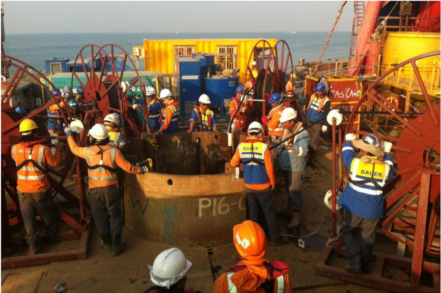
Figure 15: Shaft grouting works for the test pile
