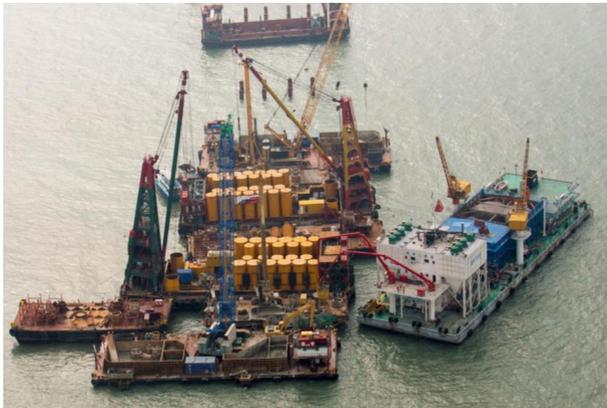
Figure 10: Pouring at the CP1 platform by Floating Batching Plant
