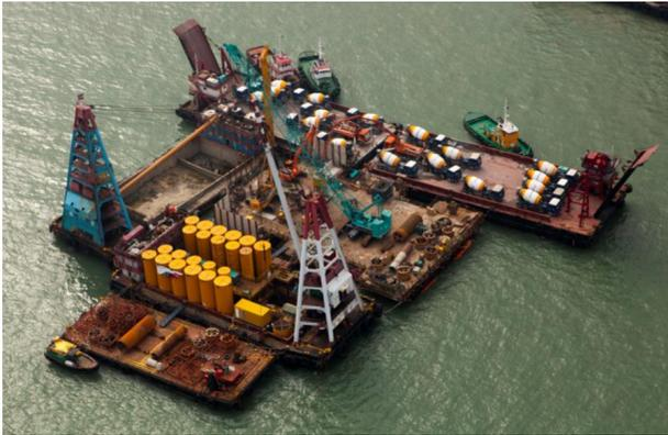
Figure 9: Pouring at the CP4 platform by RoRo-Barge with trucks
