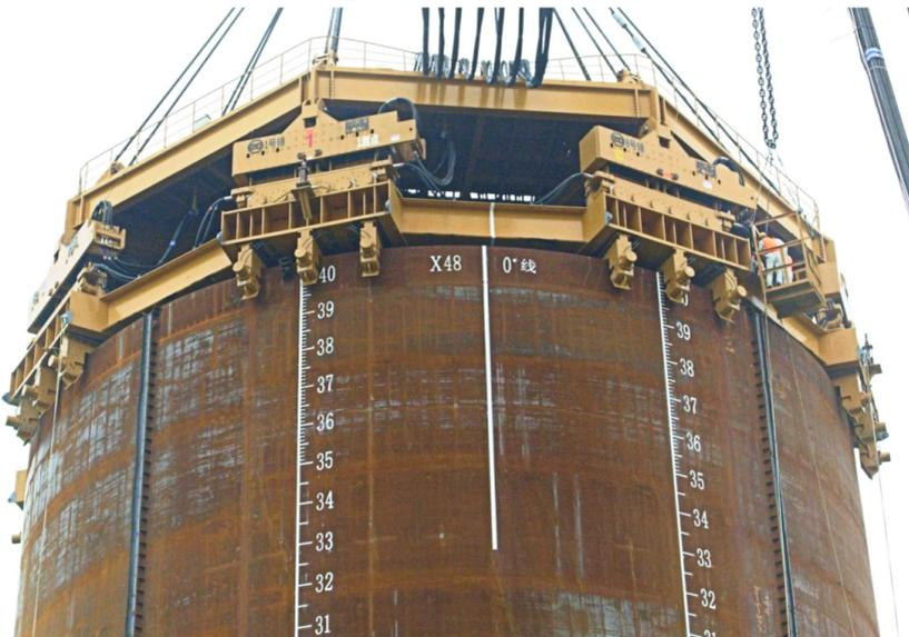
Figure 1, Vibratory driving of 22 m diameter pile in China
