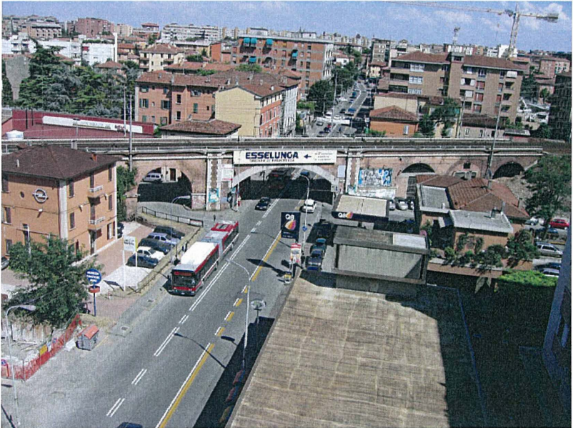
Figure 2: General view of the site with the railway bridge "Ponte Vecchio"
