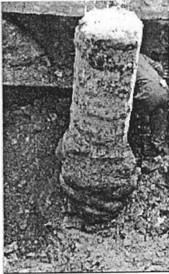
Figure 9. Cast in situ pile with bulb
