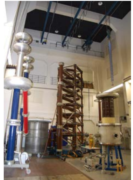
High voltage lab with vacuum vessel
