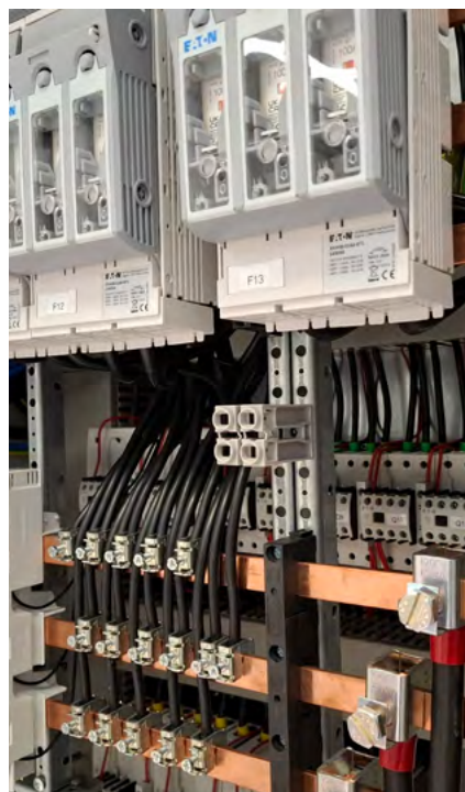
Figure 2: phase distribution via busbar system
