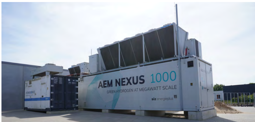
Figure 4: 1 MW AEM- electrolyzers
