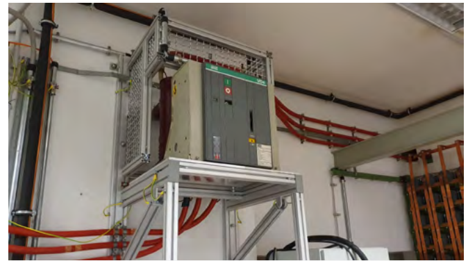
MEDIUM-VOLTAGE CONNECTION
