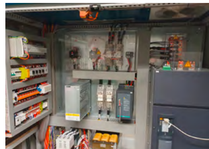
LVDC SWITCH CABINET WITH LVDC AFE & DC BUSBAR
