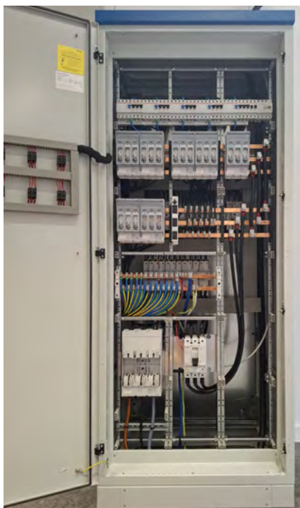
Figure 1: laboratory distribution without contact protection
