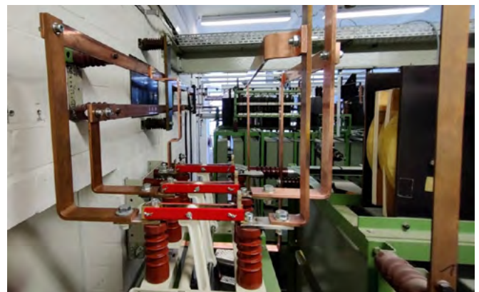
Assembly of a 6kV disconnect switch and connection via copper busbars
