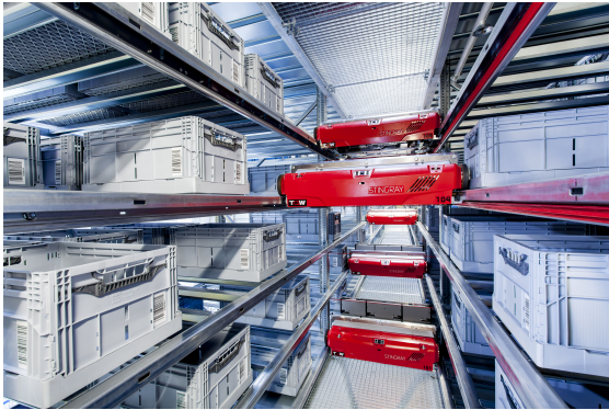
(a) Automated storage facility 3
