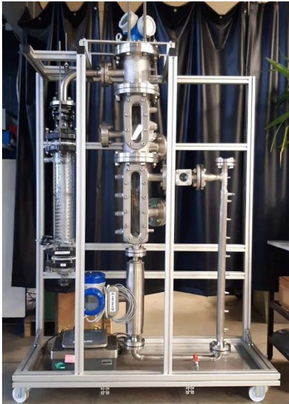
- Plant under construction -
