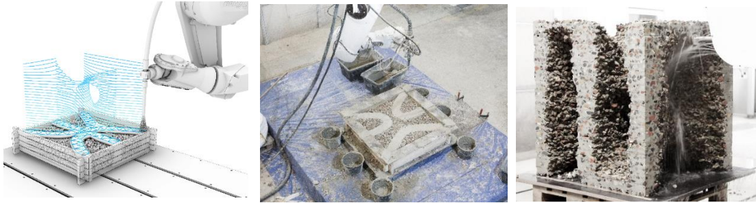
Abb. 1. Large Particle 3D Concrete Printing Verfahren im Digital Building Fabrication Laboratory
