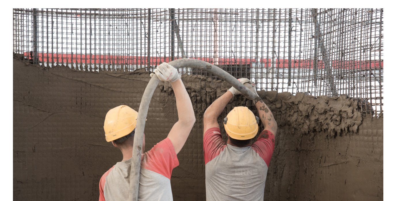
Mesh Mould, Phase 2: Filling of the mesh by manually „printing“ on and into the mesh.
